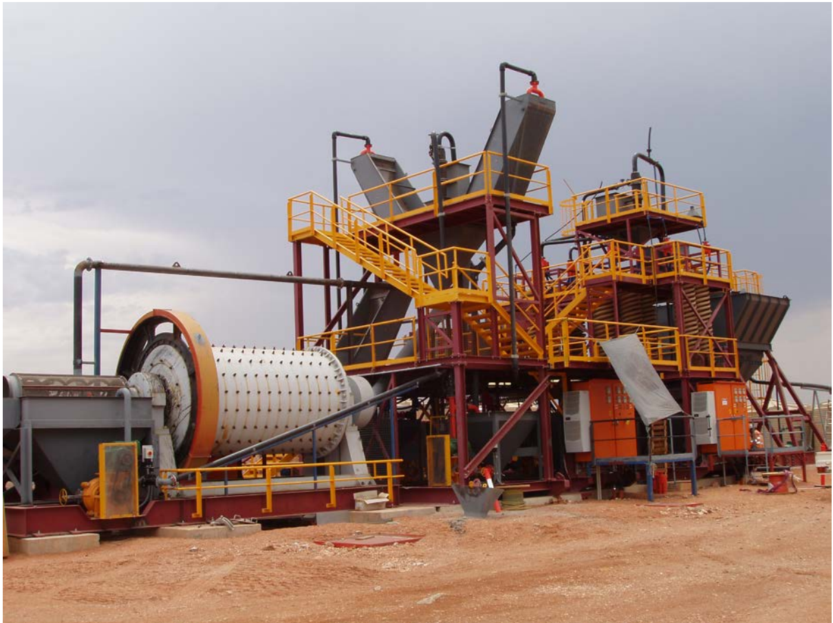
Figure 4: Tabba Tabba Plant as constructed (in-situ)
