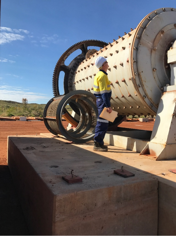
Figure 1: Ball Mill on foundations
