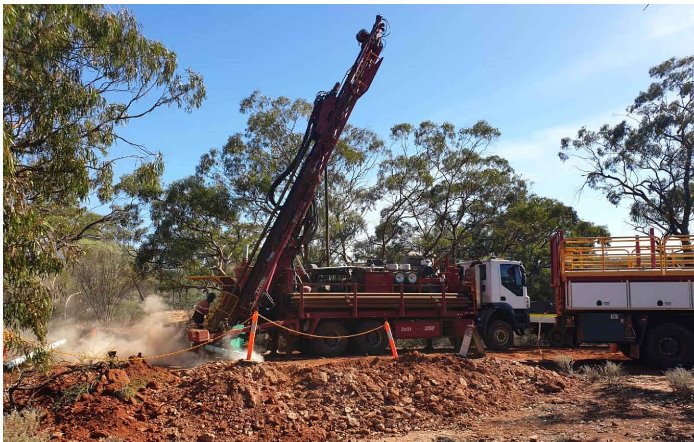
Figure 2: Drilling at the Mount Mulgine Tungsten Project
